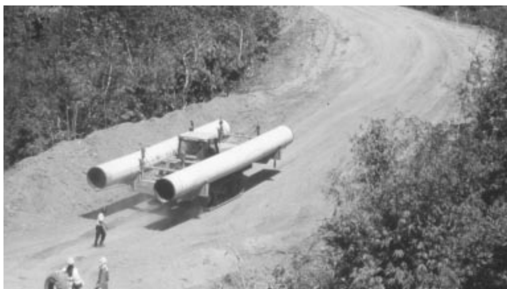
Construction of the Yadana Gas Pipeline in Thailand. (credit: Earthrights International)
